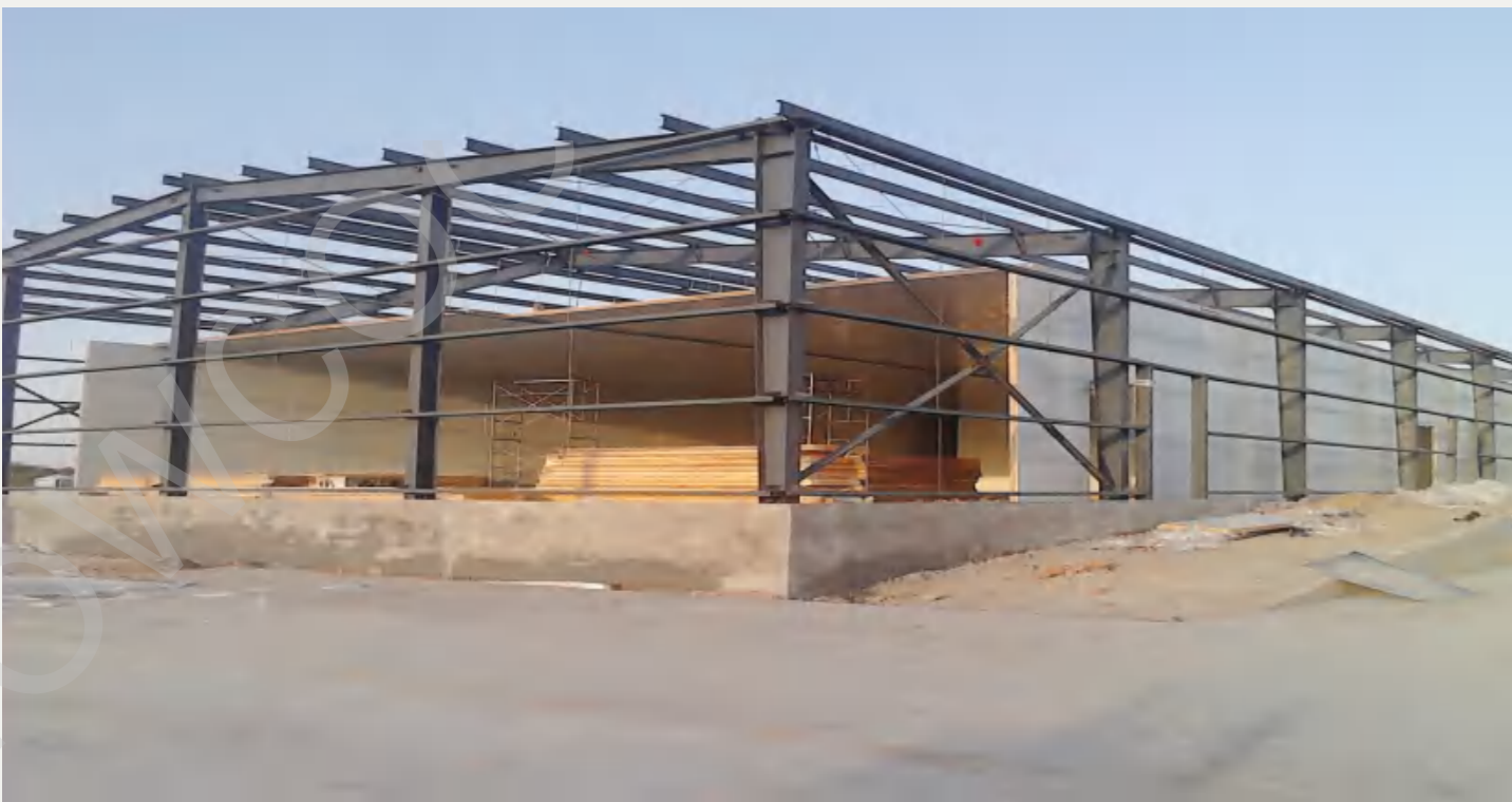
Main structure of large steel cold storage
