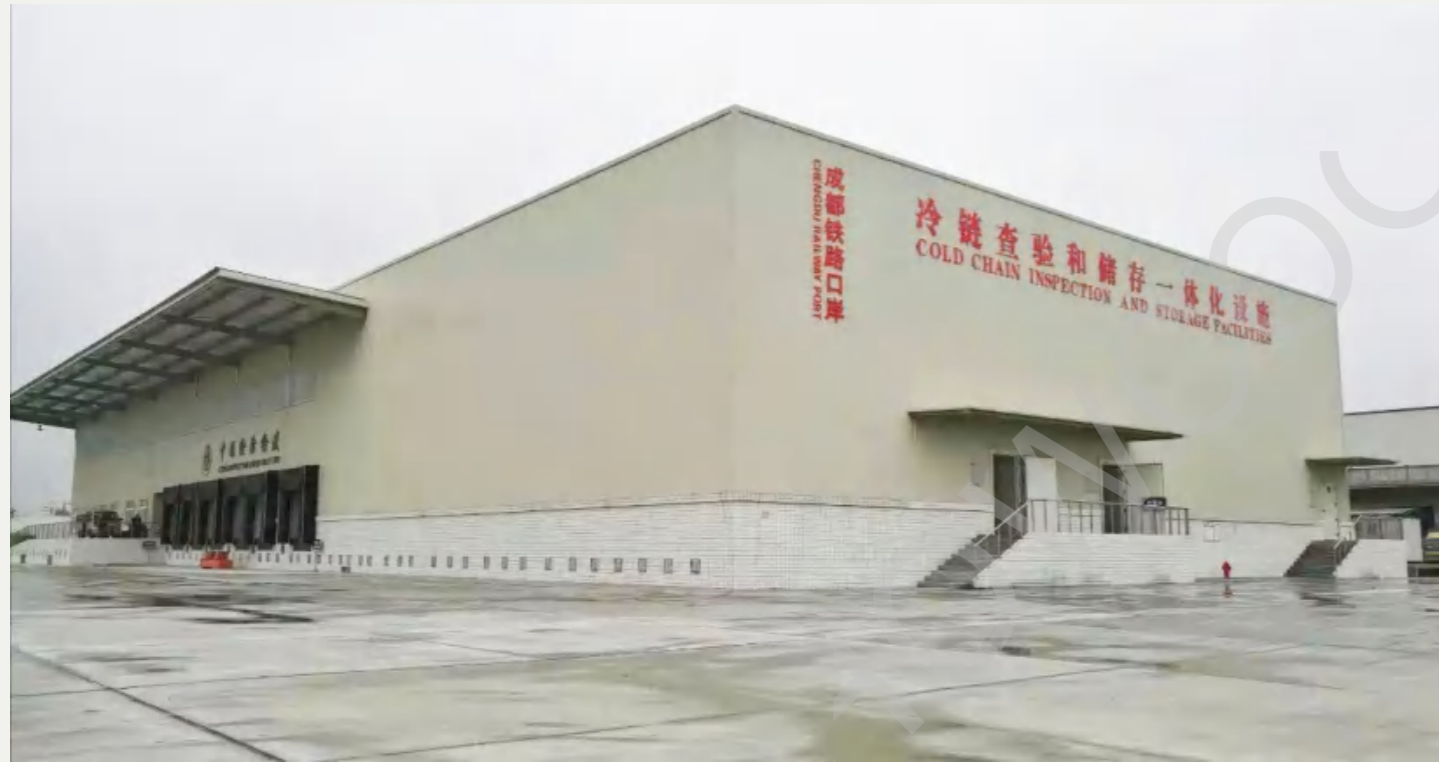
5000 ton cold storage project at railway port
