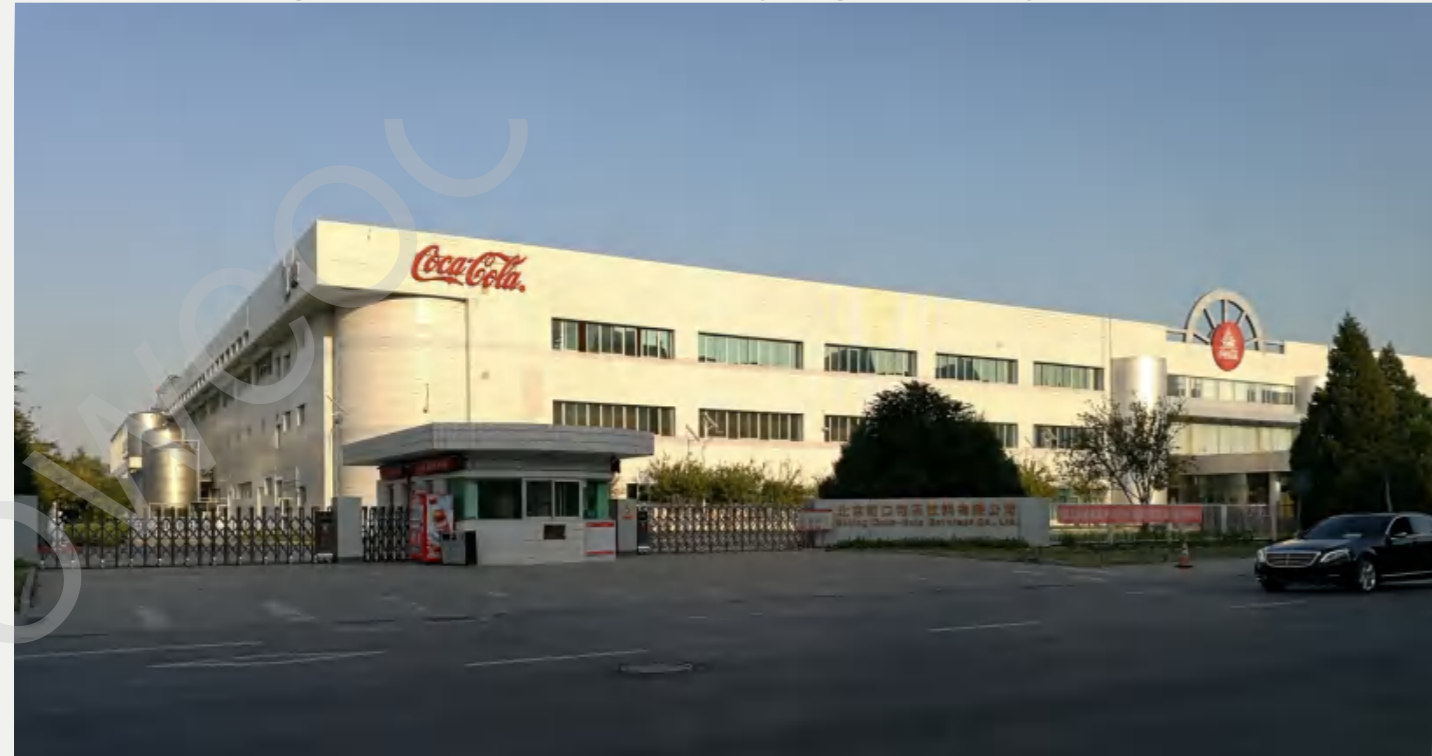
Cold storage of Coca Cola Beijing factory
