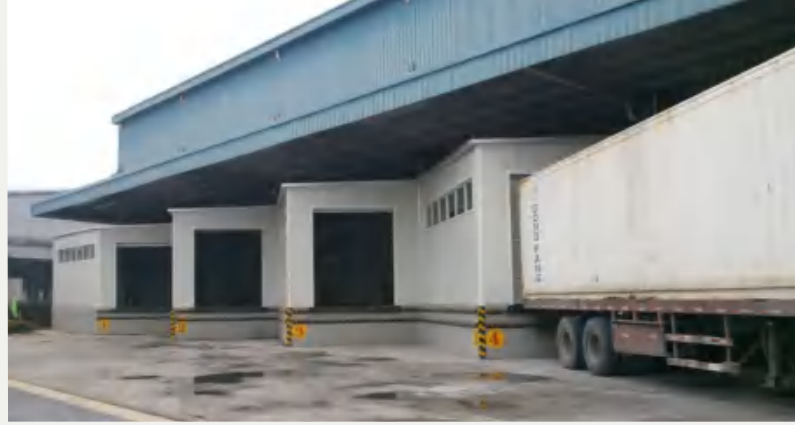
Cold storage door
