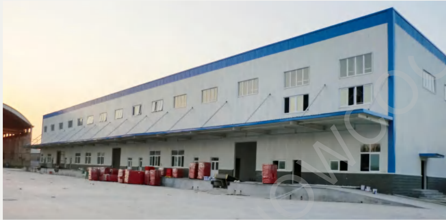
50000 m3 cold storage project
