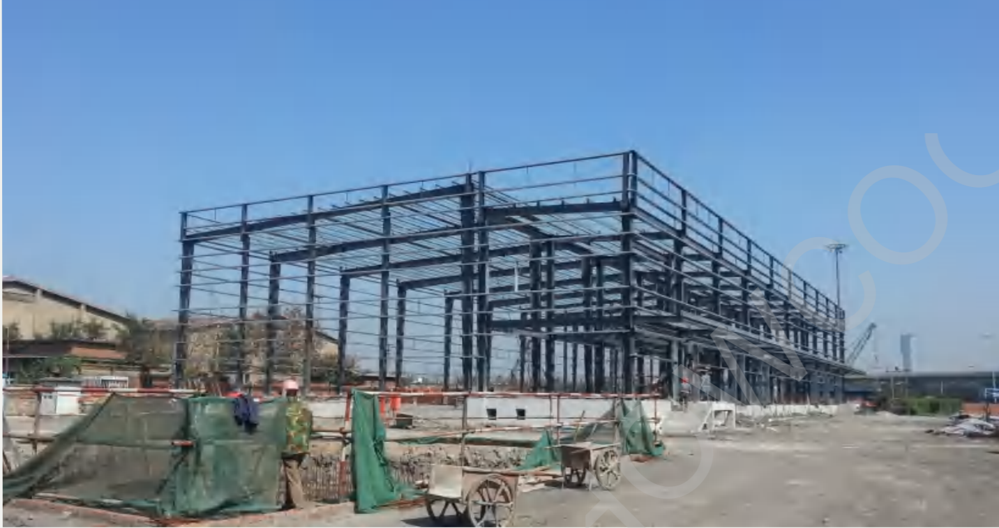
Main structure of large steel cold storage
