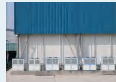
Finished Condensing Unit Installation
