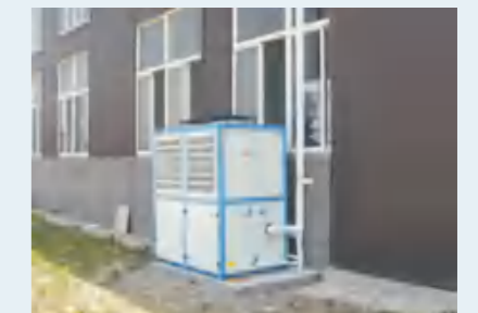
Finished Condensing Unit Installation
