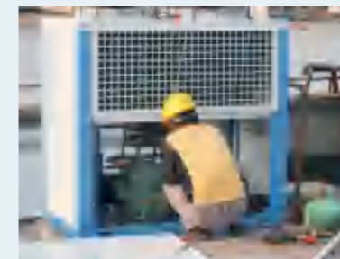
Condensing Unit On Site
